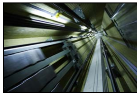
Inside the test tower. View from below in the lift shaft
