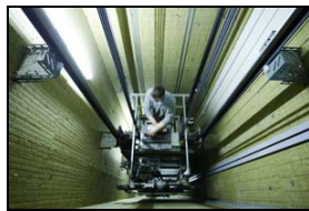
Inside the test tower during the tests
